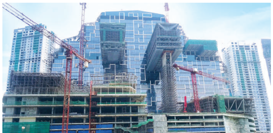
Ongoing construction at 'Cinnamon Life'
