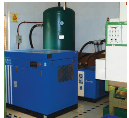
Screw compressors used at TSF factories
