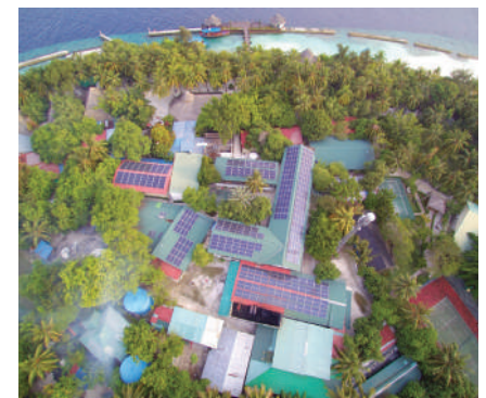
Solar panels generating renewable energy at 'Ellaidhoo Maldives by Cinnamon'
